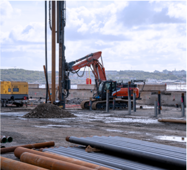
Piling work at the Skandia Port for the Skandia Gateway project.
